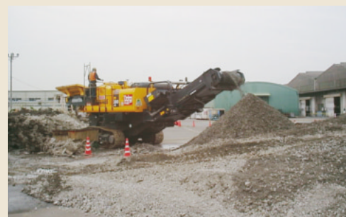
Recycling crushed concrete
