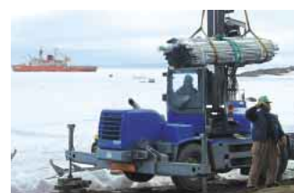
A crane powered by Isuzu diesel
