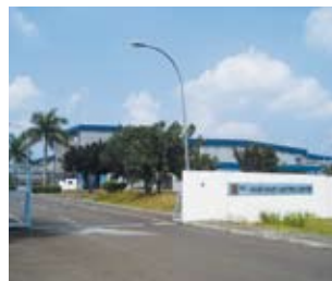
Entrance to AICC factory
