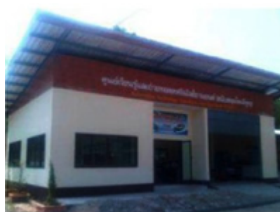
Support for foundation of an engineering transfer center at the vocational school
