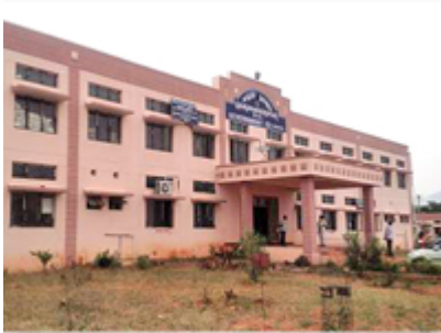
ITI school building
