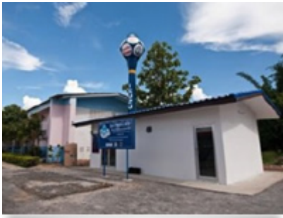
Donated clean water system building
