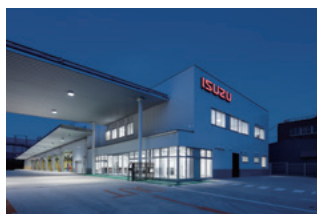
New site with LED lighting installed
