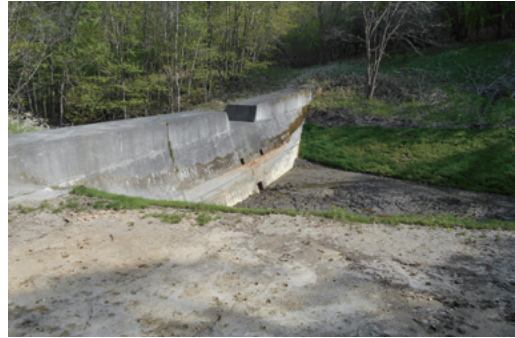
Mud-control dam installed in the site
